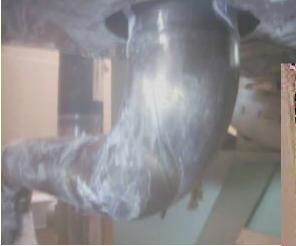
Leakage of primary coolant in the reactor containment 51 ton
