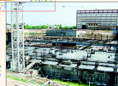
Construction site of Prototype Fast Breeder Reactor at IGCAR
