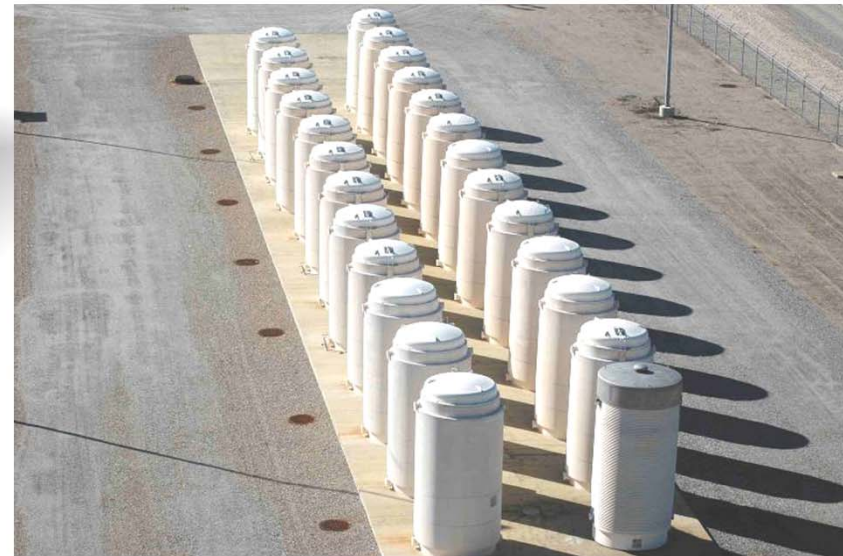
Dry Storage (Surry – USA)
