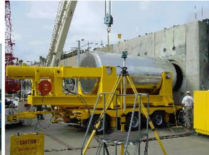
Storage of spent nuclear fuel (Baikal -1)
