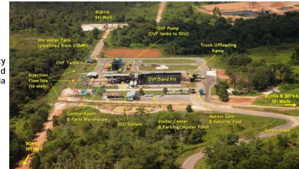
Terralog's Deep Well Disposal Best Practices adopted by the operator.
