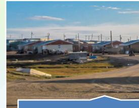
III. Off-grid communities (1 to 10 MWe)
