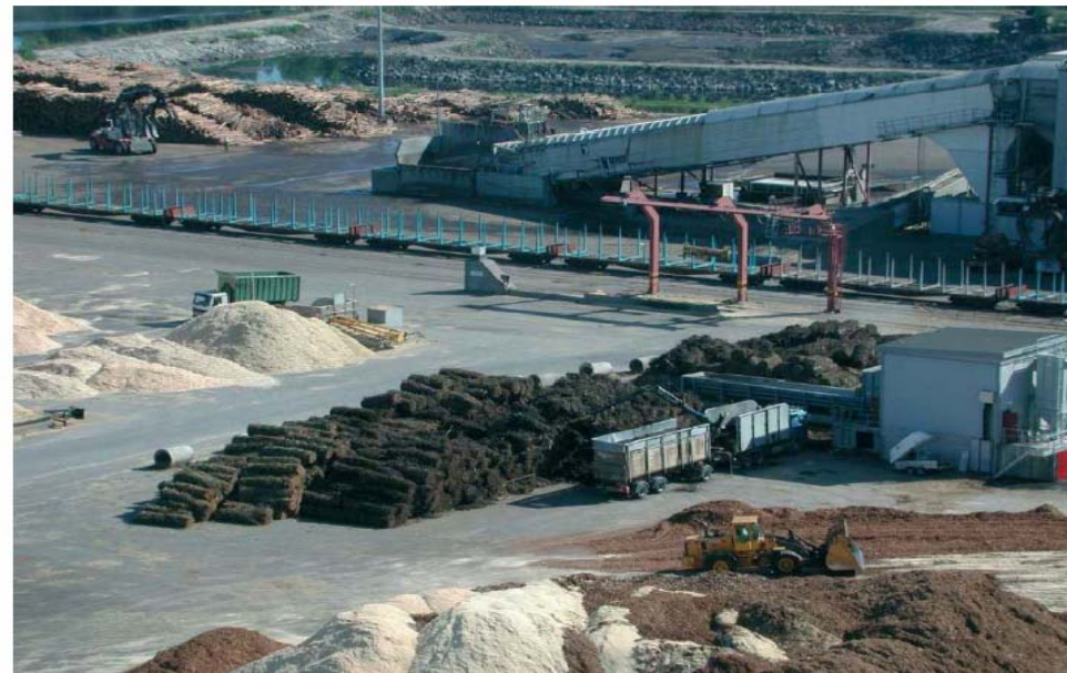
Figure 32. Compacted residue logs in front of the crushing station of Alholmens Kraft power plant (E.V.A.).
