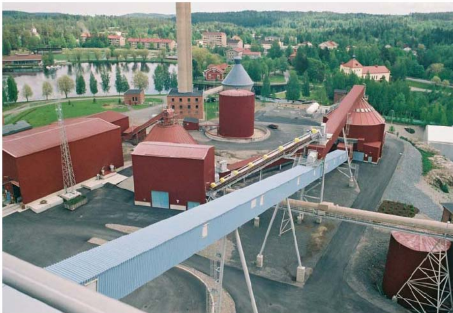
Figure 49. Fuel receiving and handling system of Jämsänkoski power plant (VTT).
