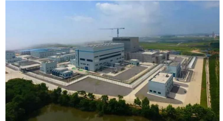
Construction site of HTR-PM
